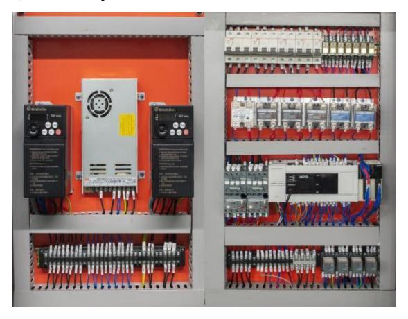
The electrical department adopts PLC system control, and the electrical control components adopt international famous brands to ensure the high efficiency and stability of the electrical system;
